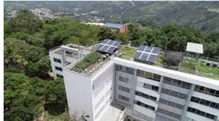
Photovoltaic system in the electrical engineering building, Universidad Industrial de Santander. Taken from http://e3t.uis.edu.co/eisi/
