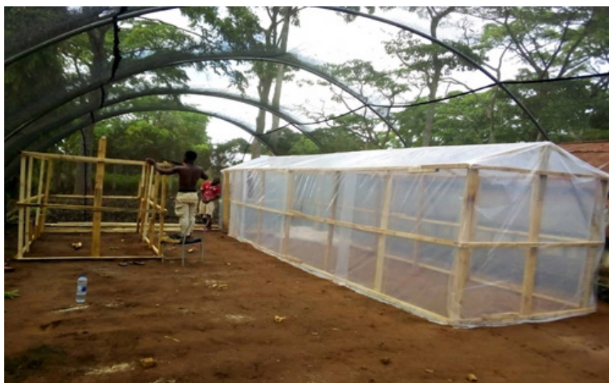
Figure 1. Construction of the sprouting and rooting chambers at TARI Naliende, Tanzania.
