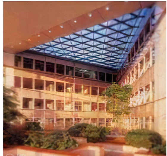
Figure 10. It shows the ventilation and lighting openings of the tower, the commercial headquarters bank –in Germany.
