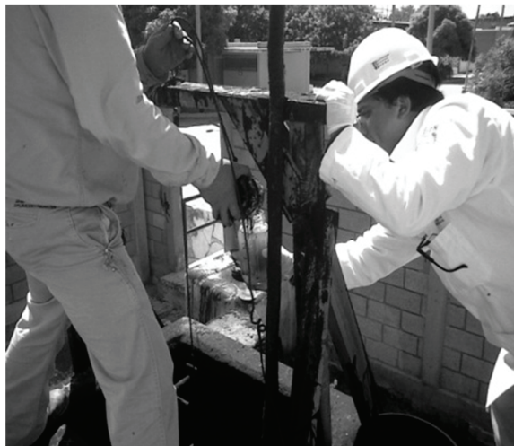
Figure 4. Injection plant, Tamaulipas-Constituciones field.
