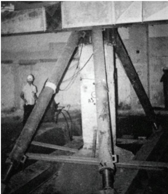
**Figure 7.** Foundation reinforcement at Paulista Mall ([2])
