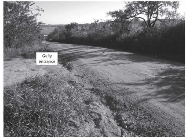
Figure 3. Cravo Stream Gully entrance, Nazareno, Minas Gerais (Brazil). The compacted road that does not have a proper drainage system can be seen. Source: The authors.
