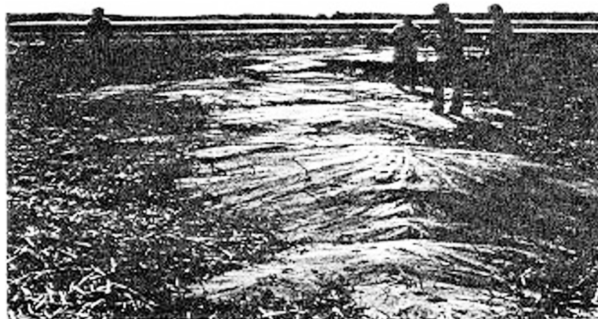
Figure 1. Sand boils due to the liquefaction phenomenon at Chlef region
