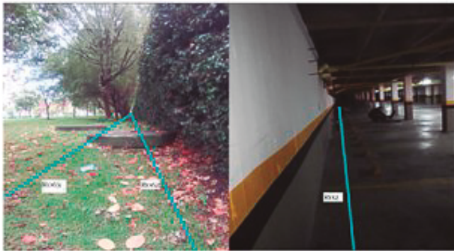
b) GPR Acquisition lines next to the retaining wall
