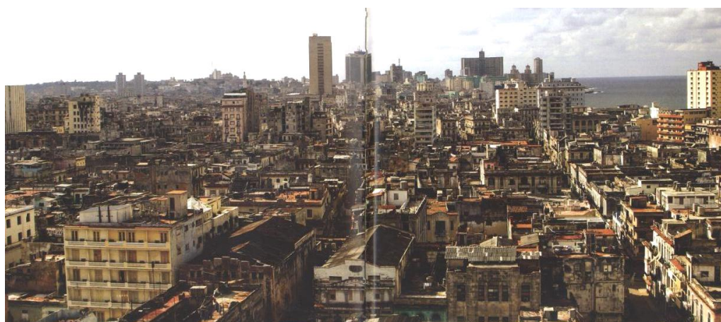
Figure 5.1 Aerial view. Existing delapidated colonial and modern buildings
