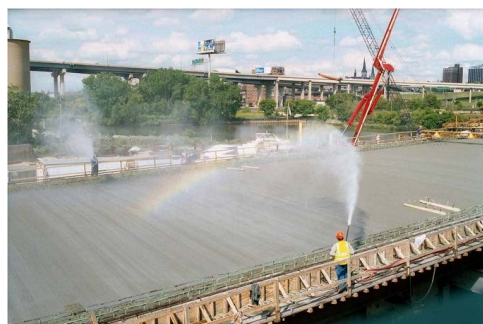
Figure 1. Concrete external curing.
