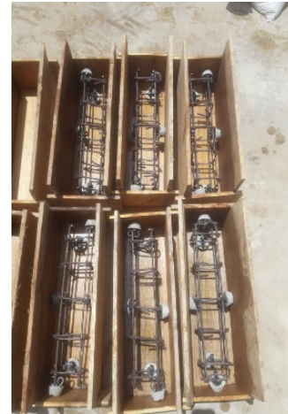
Figure 2. Joist reinforcement.
