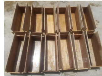
Figure 1. Joist formwork.
