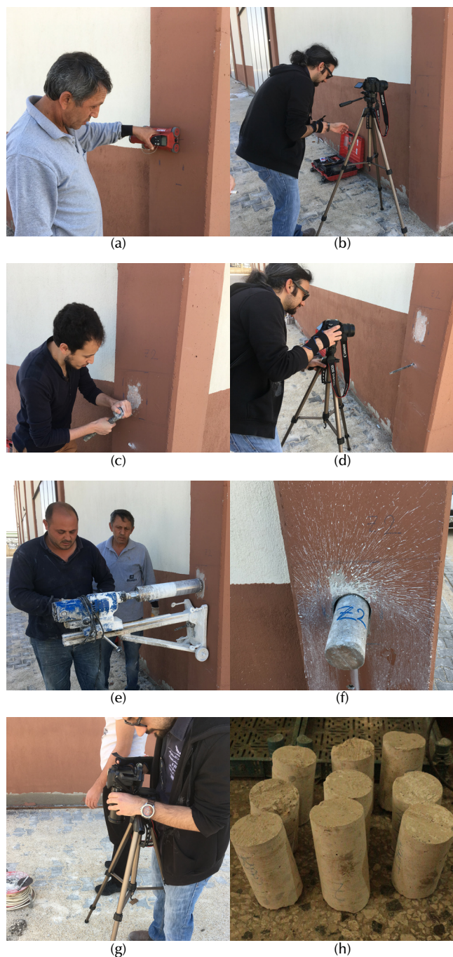
Figure 6. Coring from buildings and imaging of cores Source: Authors
