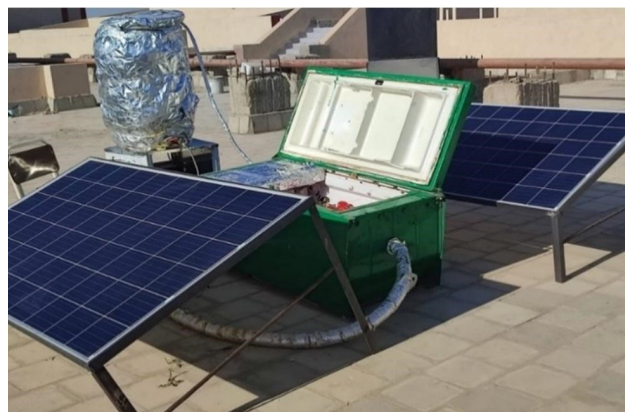
Figure 1. The indirect evaporative solar pre-cooler (IESP) experimental setup.
